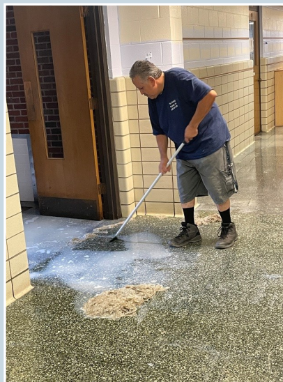
After one scraping, a noticeable difference can be seen!
