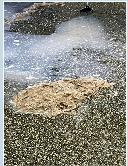
This is the wax that was scraped off from the first scraping (from just a small area of the floor.)
